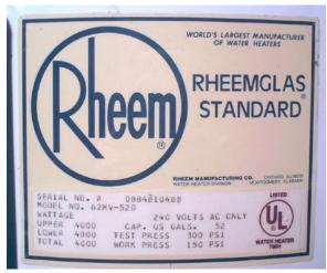
Manufactured in August 1984, 50 gallon electric, equipped with 4000 watt elements.
